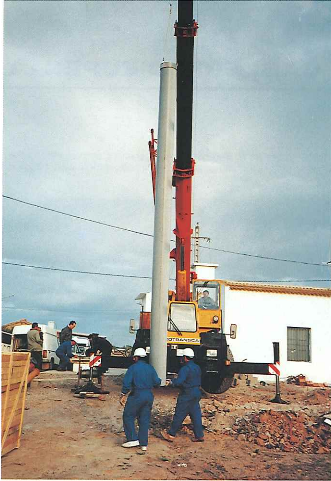
Fig. 10: Mounting of an SFCD-plain pipe element.
